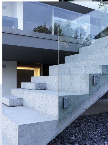
PRECAST CONCRETE STAIRCASE USE OF BATTENS & GLASS BALUSTRADE
